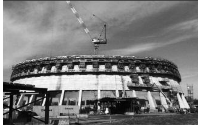
The first Cooling Tower at Brayton Point approaches 100 feet on its way to 500 feet.
