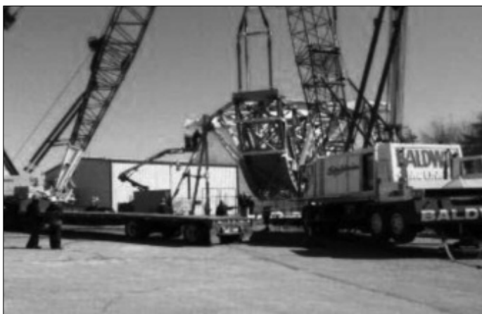
Baldwin Crane making a twin pick of a satellite base at MIT in Westford, MA
