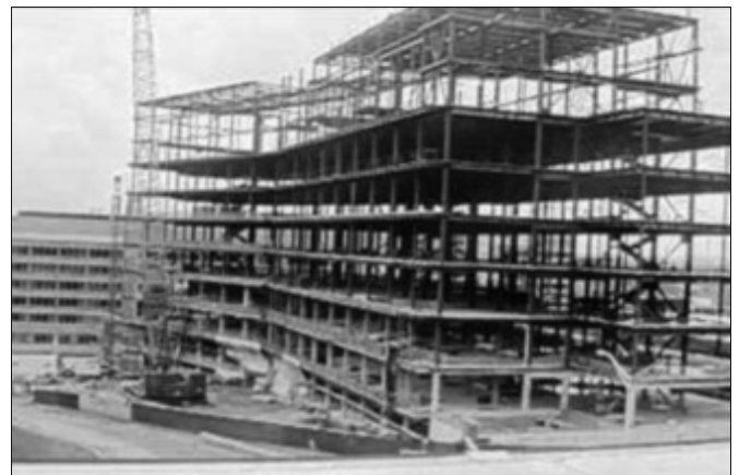
Brother Joseph Flammia and Apprentice Matt Cole are on the M-250 setting iron for J.F.Stearns at the New Albert Sherman Center in Worcester.
