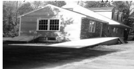
The Theodore residence after addition and new driveway.
