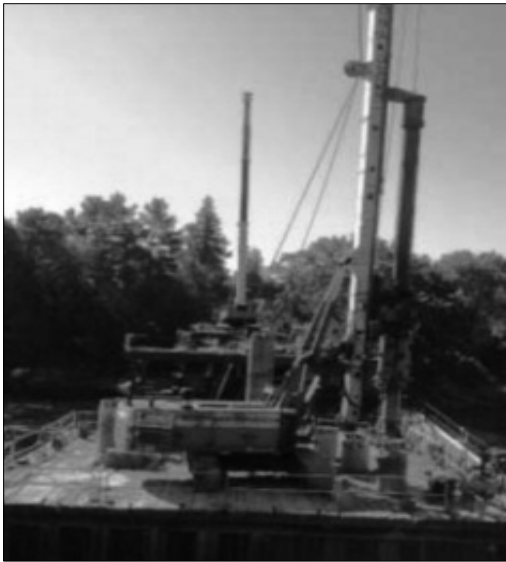
Donaldson's drill rig on Barletta's Hynes Bridge job in Amesbury
