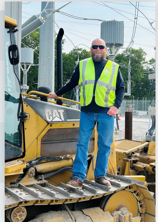
Jimmy Waugh working for Camputaro in Leicester at a new substation.
